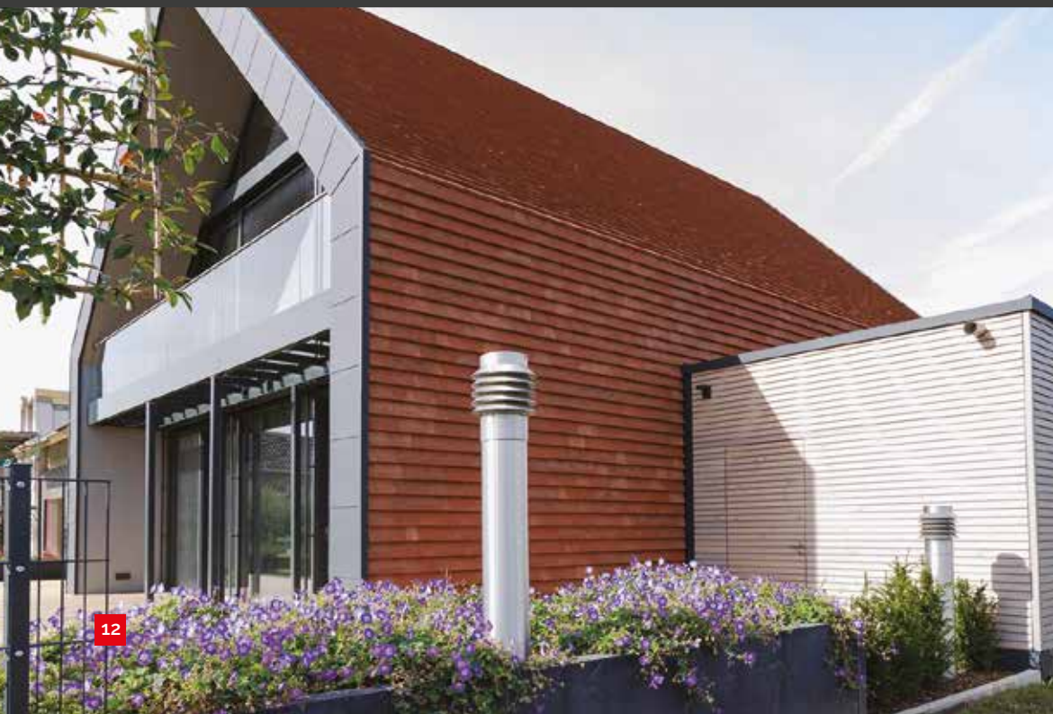
CREST NORDIC Rust Red Innovation house Terhalle Holzbau, Ahaus, Germany
